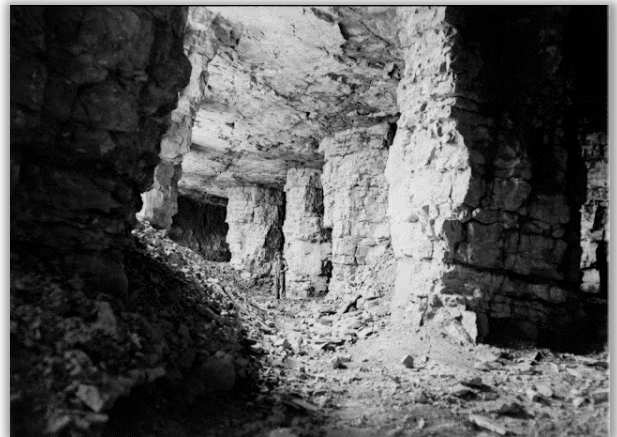
Pillar and stall mining of limestone, Gorebridge, 1945. Source: BGS
