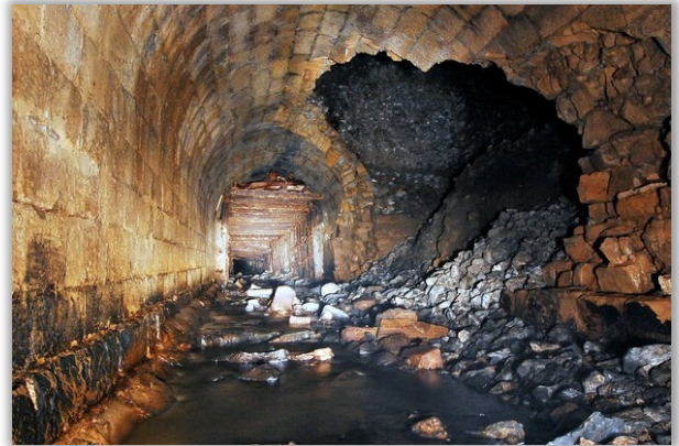
Grinkle ironstone mine culvert collapse, North York Moors
