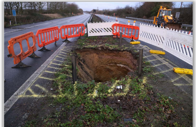
Void in central reservation of M2 due to a chalk mine. Source: Highways England
